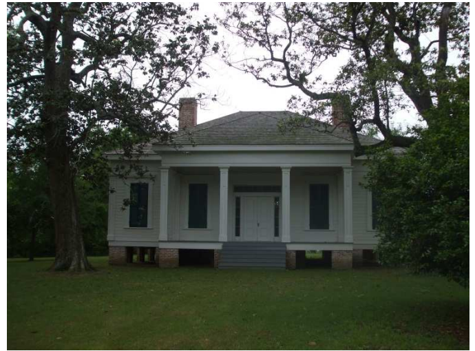
The Coker house built 1838 (?). In progress of being restored. Several miles from the hill.
